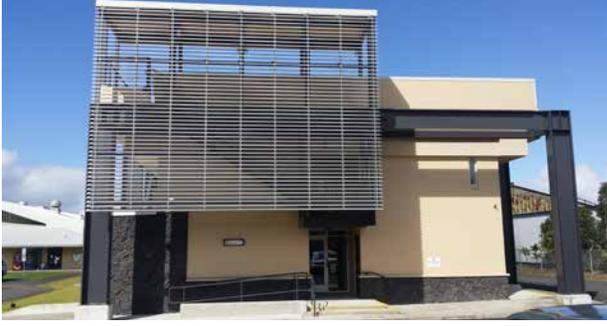
**BUILDING REUSE:** Hale Aloha reuses over 67% of the existing building shell including existing exterior concrete and CMU walls, structural concrete floors and slabs, thereby reducing construction demolition waste in landfills and the use of new materials.
