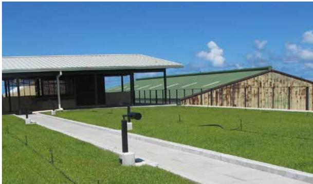
**GREEN ROOF:** Hale Aloha's new roof is supported by steel columns. The roof has 5,490 SF of accessible vegetated roof - which activates the space and contributes to stormwater management. The green roof absorbs and retains more water on site than a typical metal roof that creates stormwater runoff. The green roof also provides additional insulation for the building, keeping it cool on warm days and saving energy needed to run the A/C.
