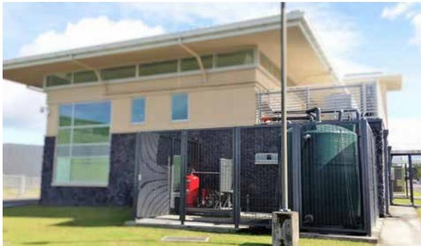
**RAINWATER HARVESTING:** The annual rainfall in Hilo, HI averages 134 inches. To take advantage of this water source, Hale Aloha has a rain cistern that captures on average 144,000 gallons of water from the roof per year. All of the toilets and urinals in the building are flushed using captured rainwater.
