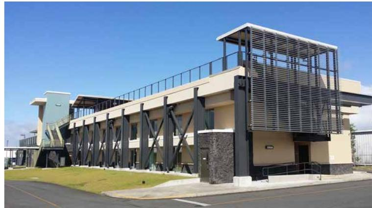
**THE GREENEST BUILDING IS AN EXISTING ONE:** The design for the renovation of Hale Aloha kept as many interior walls as possible and over 67% of the structural CMU walls and concrete floor slabs were left untouched. This reduces landfill waste associated with demolition.
